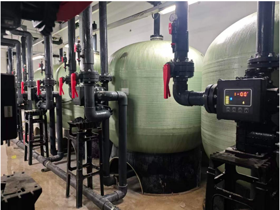
70m 3 /h Automatic Control Valve F153 Applied in Data Center Cooling Circulating Water System
